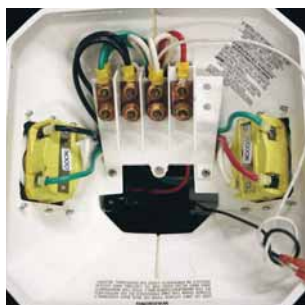
Copper Busbar with Ratings up to 140 A
